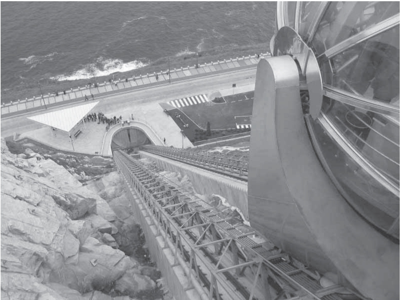
Inclined elevator A Coruña
